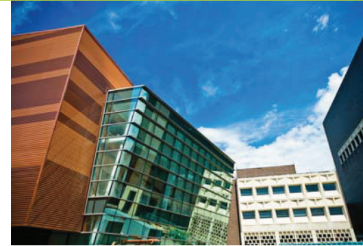
EE's home, Barbara and Jack Davis Hall
