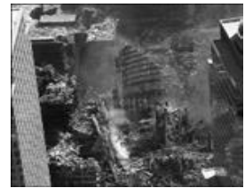
Remains of the steel frame of One World Trade Center
